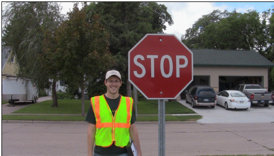
Figure 4.36 Inappropriate height of stop sign
