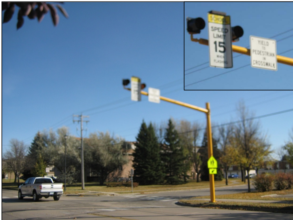
Figure 4.4 Worn out pedestrian crossing and malfunctioning speed limit sign (inset)
