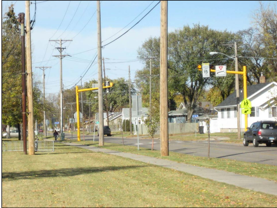
Figure 4.25 Pedestrian flashing beacons at N 20 th St and 6 th Ave N
