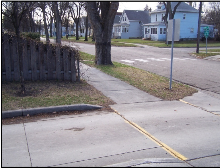
Figure 5.3. Sight Obstruction at the West Exit of the South Parking Lot
